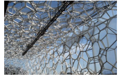
Figure 4.11 The structure of the Water Cube under construction (source: Carfrae, 2007).
